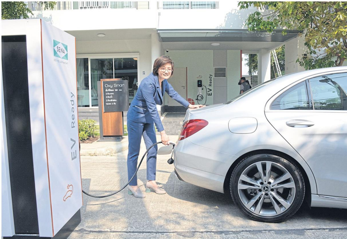
Sena Development deputy chief executive Kessara Thanyalakpark uses an EV charging station at one of the company's residential projects.
